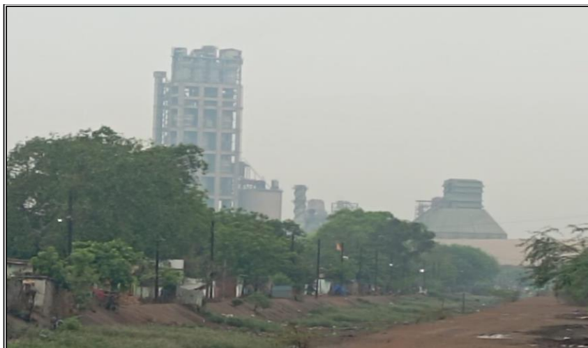
Figure: 1. Khursipar, Power House, Bhilai, Dist. Durg (C.G.)
